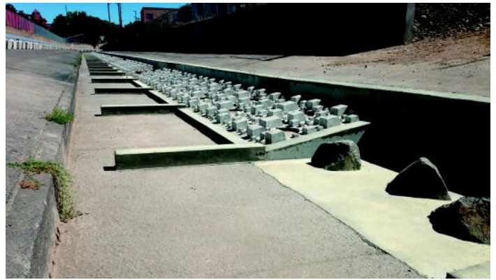
The completed channel, showing roughness panels, new baffles, and a resting pool.
