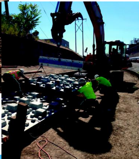
The existing concrete is cut and removed to make room for the roughness panels (above and right). Then concrete is poured in place to re-seal the channel (below).
