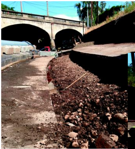
The existing concrete is cut and removed to make room for the roughness panels (above and right). Then concrete is poured in place to re-seal the channel (below).
