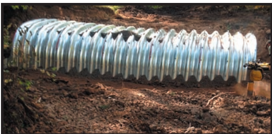
In addition to the culvert being undersized, the plunge out of the culvert was a passage barrier (above). The new arch culvert was assembled in place, shown below during backfilling. The completed structure (right) provides plenty of room for expected peak flows, and a natural stream bottom to fish swimming through.
