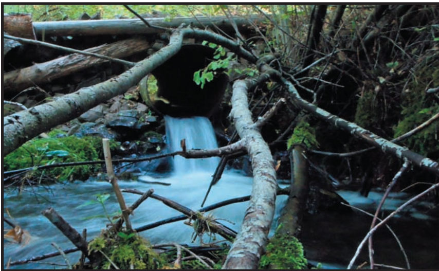
In addition to the culvert being undersized, the plunge out of the culvert was a passage barrier (above). The new arch culvert was assembled in place, shown below during backfilling. The completed structure (right) provides plenty of room for expected peak flows, and a natural stream bottom to fish swimming through.
