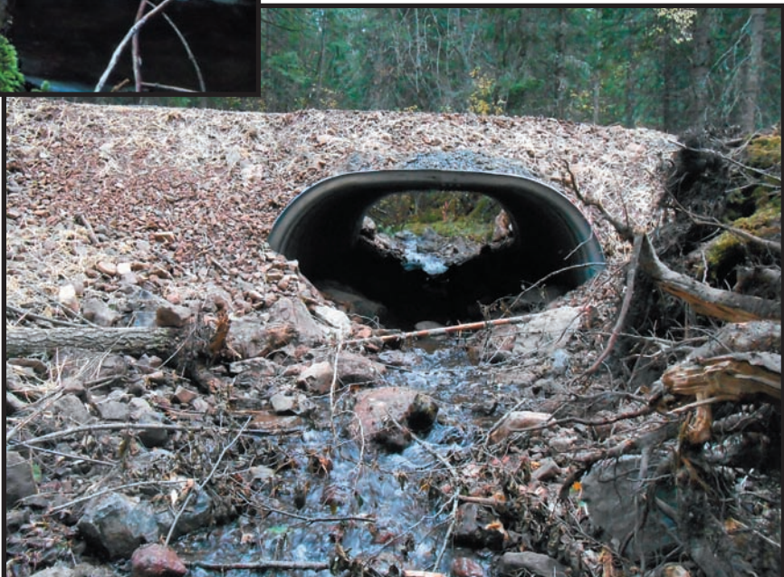
In addition to the culvert being undersized, the plunge out of the culvert was a passage barrier (above). The new arch culvert was assembled in place, shown below during backfilling. The completed structure (right) provides plenty of room for expected peak flows, and a natural stream bottom to fish swimming through.
