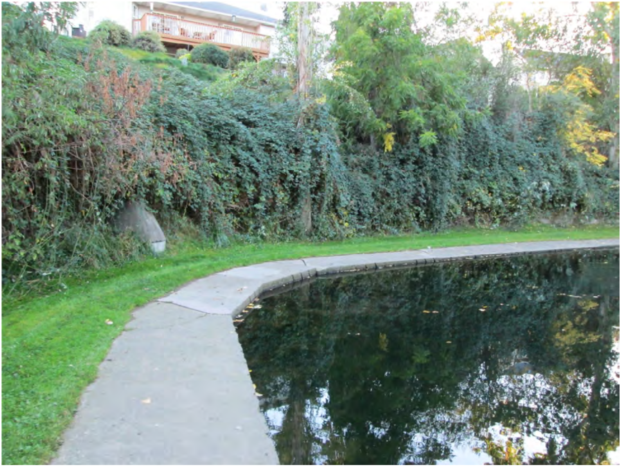
Photo 5. Stormwater inlet pipe to the fishing pond.
