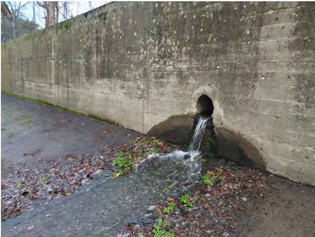
Photo 14 – 12" Drain Pipe
