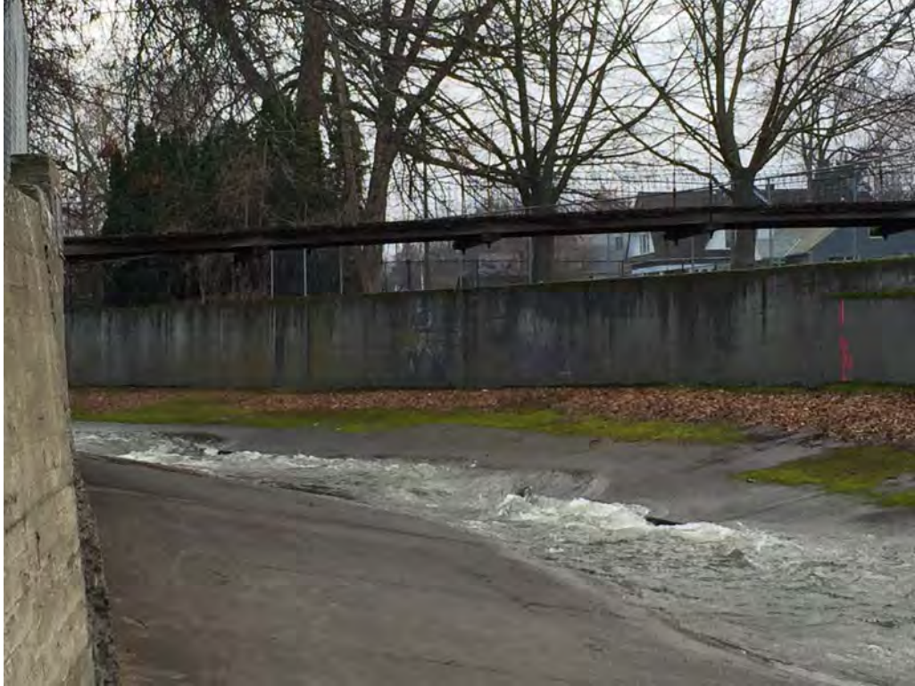
Photo 3 – Pedestrian Foot Bridge at STA 68+00.
