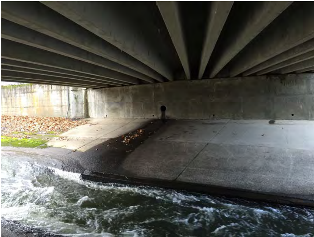
Photo 16 – Under Division Street Bridge
