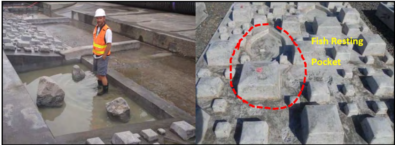
Figure 21 - Photo of fish passage elements: baffles, resting pools, and fish resting pockets within roughness panels.
