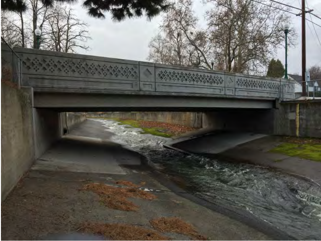
Photo 15 – Division Street Bridge
