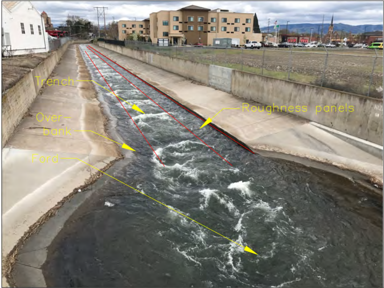
Figure 18 - Photo of baseline and modified Mill Creek channel downstream of 6th Street. The red lines in the photo are of the modified channel (right) denote the 5- to 6-foot wide fish passage corridor created by the roughness panels, V-occupied of the fish passage pathway.
