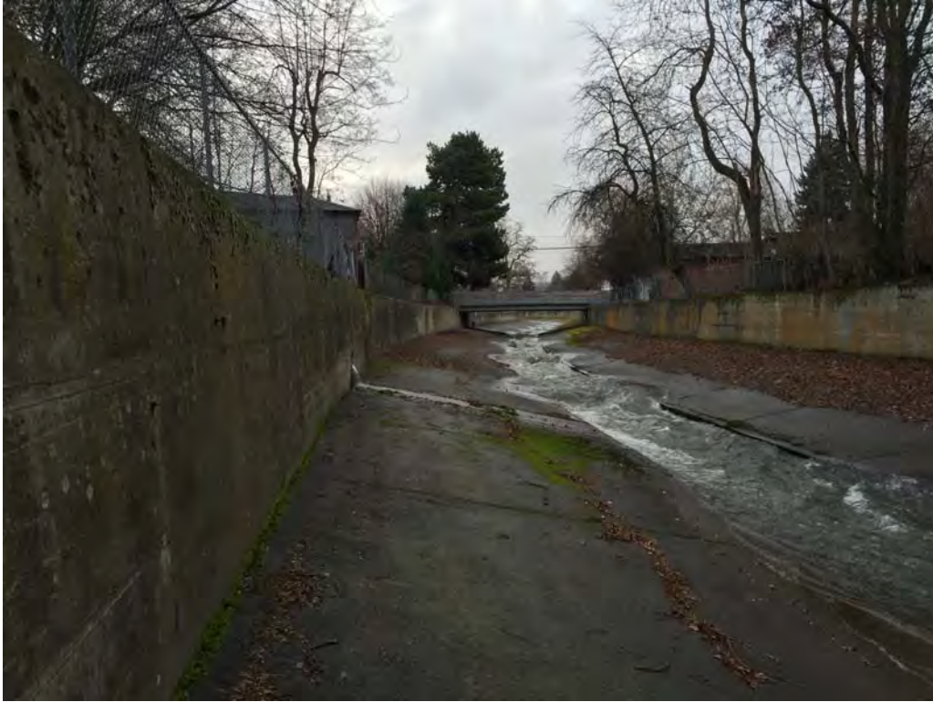
Photo 13 – View upstream of Division Street Bridge.
