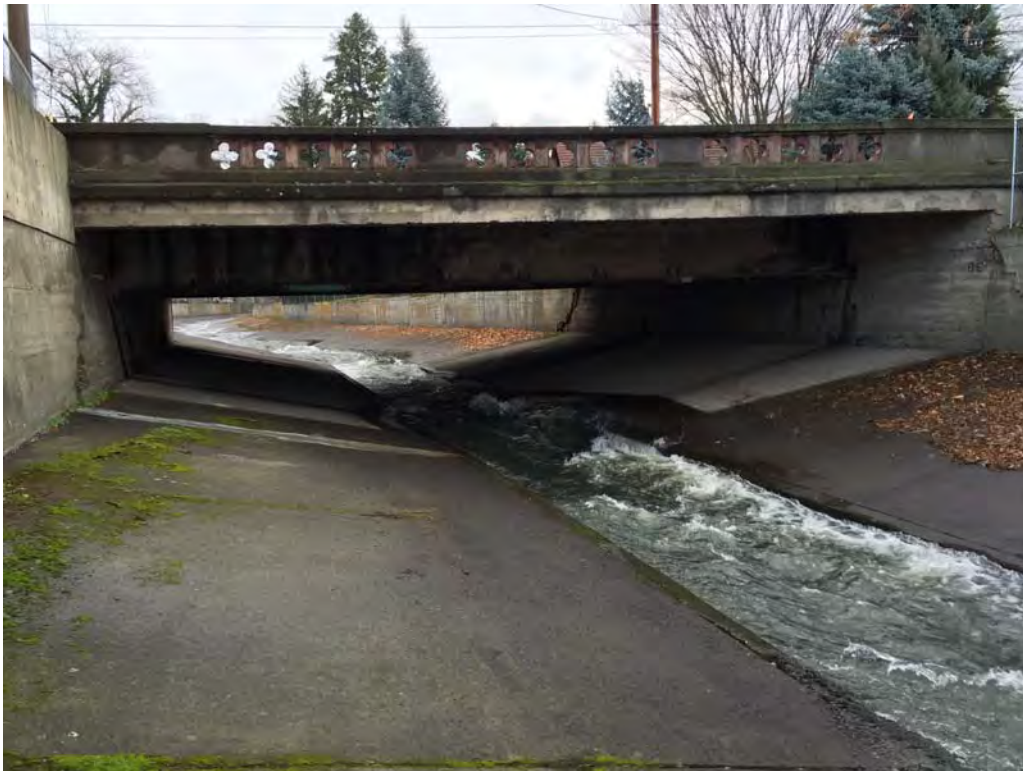
Photo 10 – Clinton Street Bridge (104 cfs).
