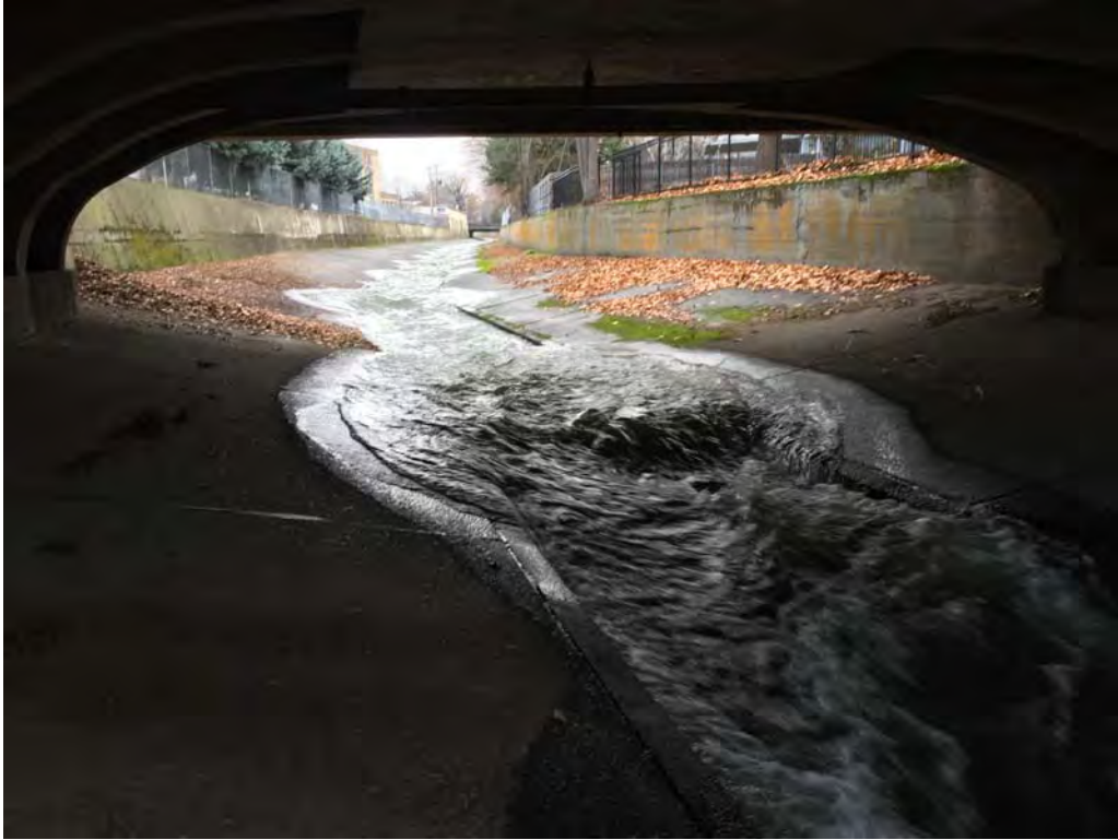
Photo 7 – Upstream View under Merriam Bridge
