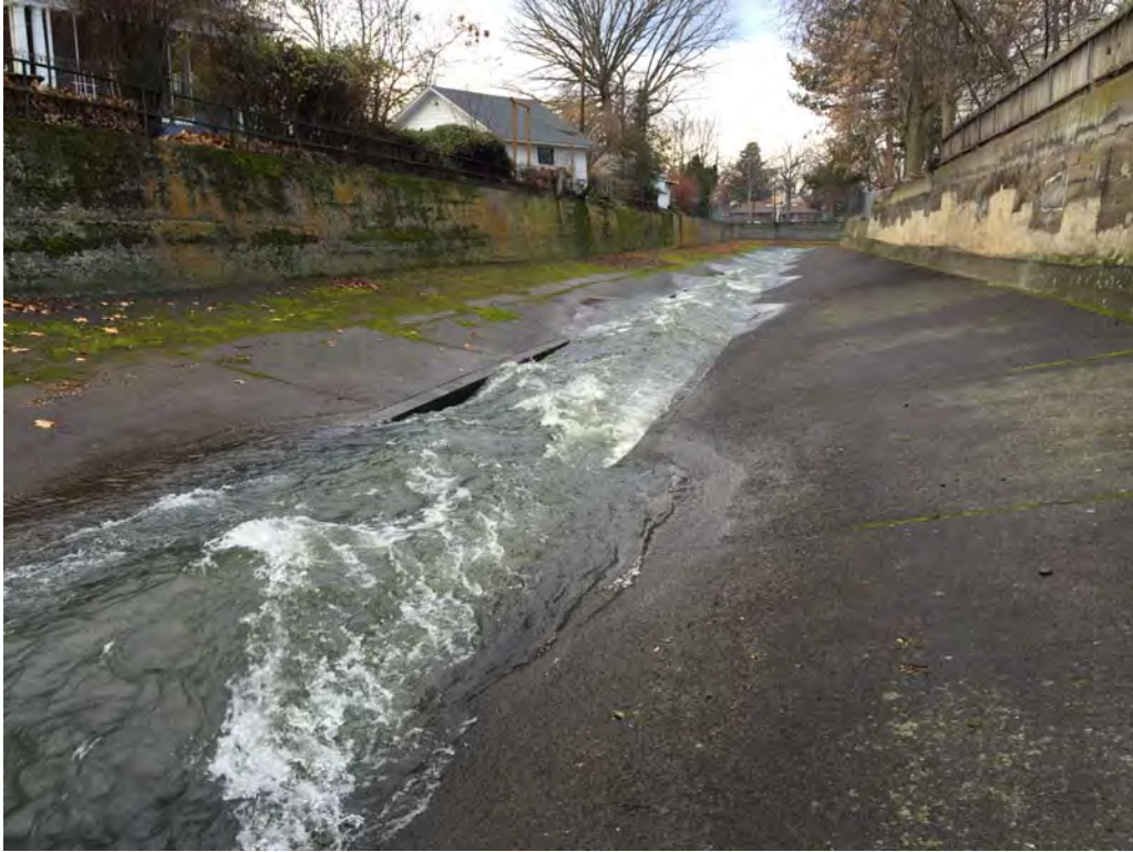
Photo 5 – Channel Downstream of Otis Street
