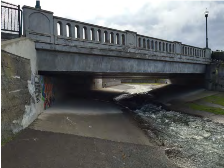
Photo 1 – View downstream of Park Street Bridge.
