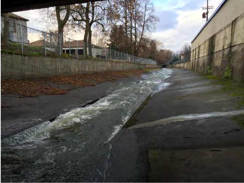
Photo 11 – View downstream towards Merriam Street Bridge.
