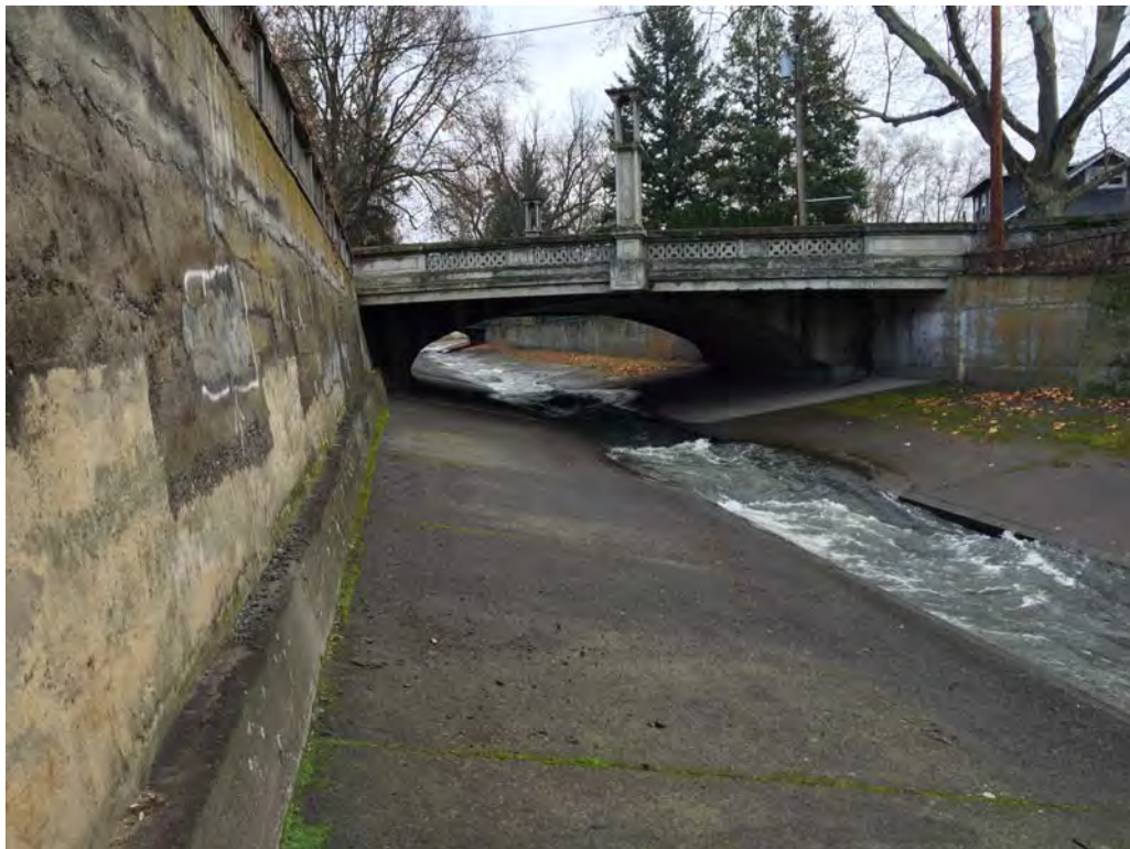
Photo 4 – Upstream View of Otis Street Bridge (104 cfs).
