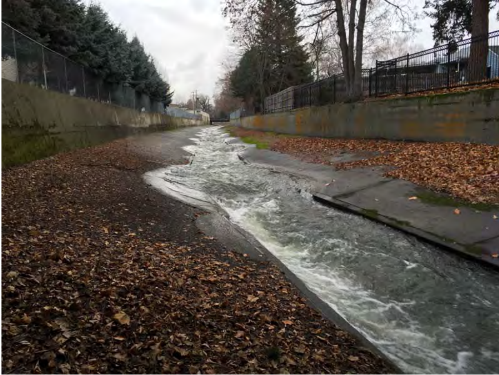
Photo 9 – View upstream towards Clinton Street Bridge (104 cfs).
