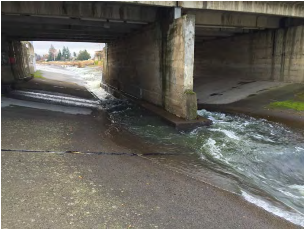
Photo 19 – Roosevelt Street Bridge
