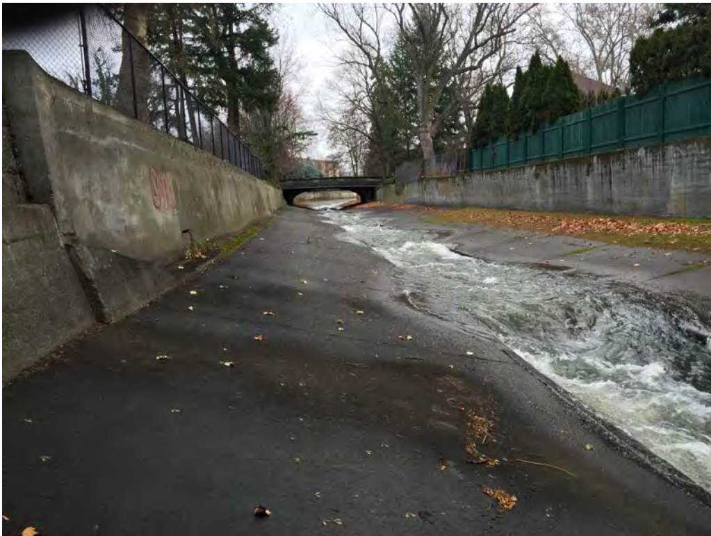
Photo 6 – Upstream view towards Merriam Road Bridge.
