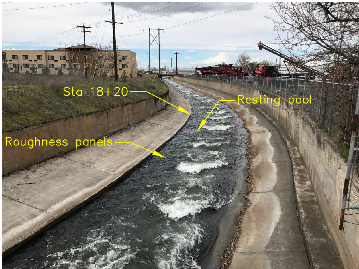
Figure 20. Photo showing the “sweet spot” for fish passage as a continuous pathway for fish to swim upstream along the left side of the channel. The “V-occupied” fish passage pathway area is clear along the left margin of the streamlines where the water depth varies from ~1’ to 3’ over the roughness panels and resting pools. Flat flow is a little more nuanced where the resting pools exist but can be seen at the arrow and the resting pool downstream.
