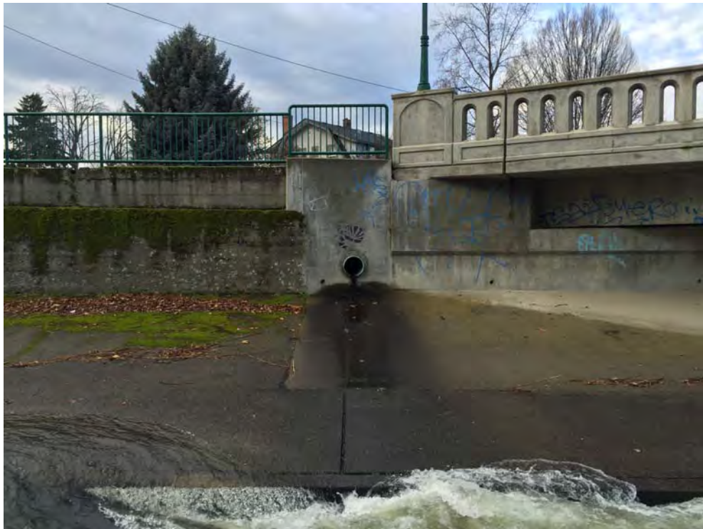
Photo 2 – Stormwater outlet upstream of Park Street.
