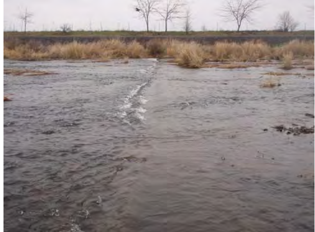
Photo 7-5: Reach Type 1 Segment E Depositional Area – Sill is partially buried from gravel accumulation.
