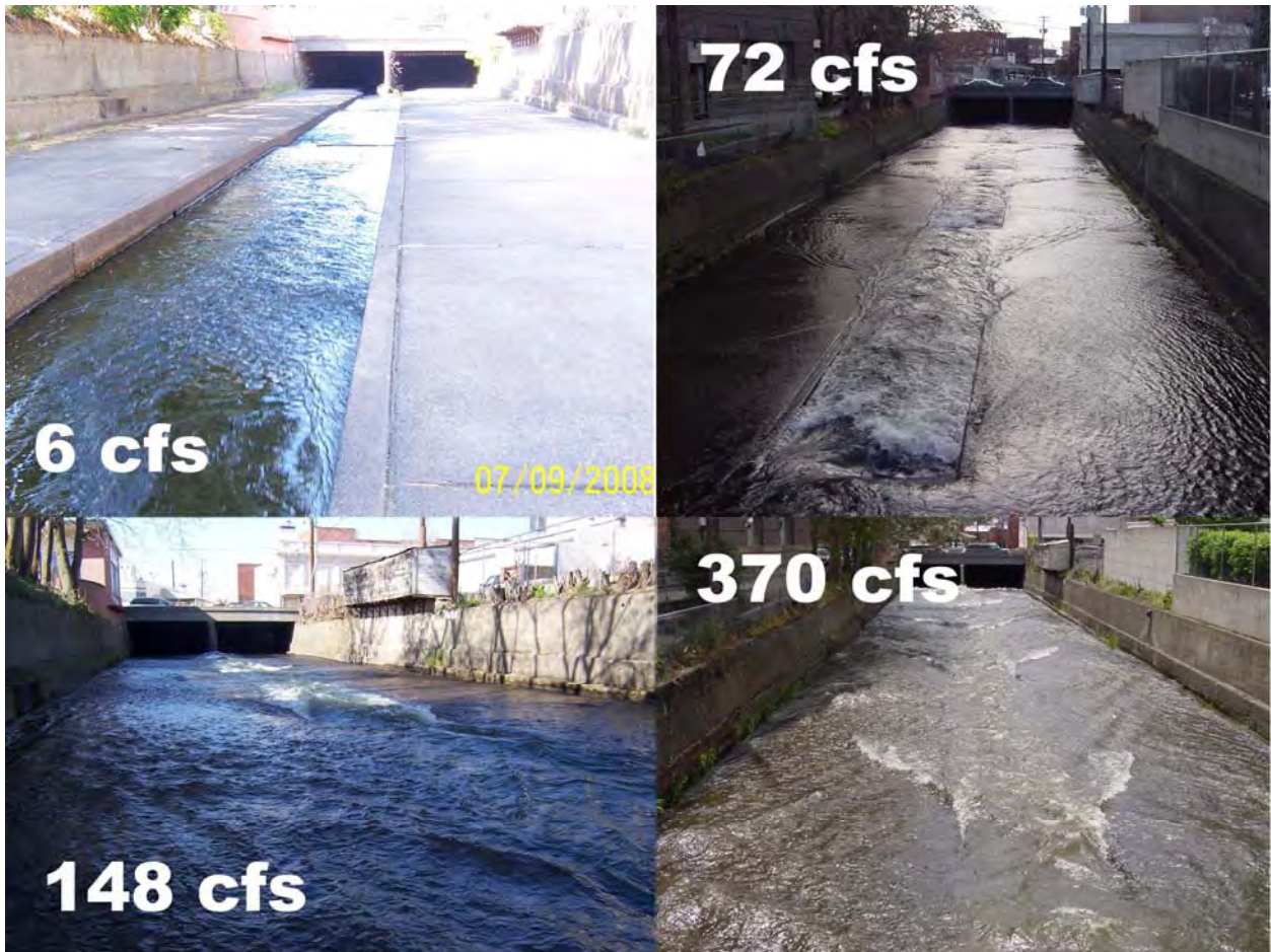
Photo 5-1 – Reach Type 6 at flows of 6, 72, 148 and 370 cfs. View is downstream with Colville Street in the background. Depth in the overbank area at 148 cfs is 0.3 to 0.4 feet.
