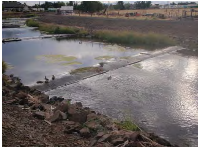
Photo 7-2: Reach Type 1 Segment B Concrete Sill. Flow is 5 cfs.
