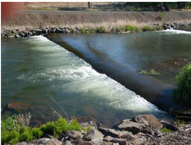
Photo 7-6: Reach Type 1 Sill in Segment F (above Tausick Way).
