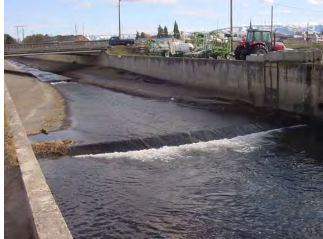
Photo 2.2 – Upstream View of Reach Type 2 Flume Transition at 27 cfs.
