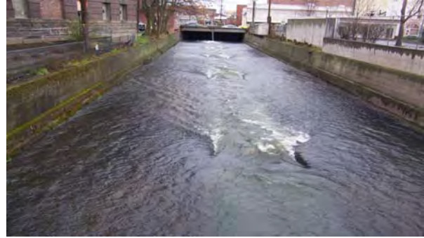
Photo 2.5 - Reach Type 6 at 208 cfs. The start of underground section is visible downstream. View Downstream.
