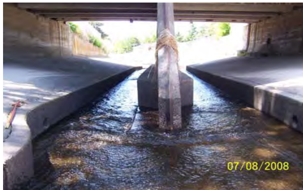
Photo 2.8 - Reach Type 10 Roosevelt Street Bridge Pier. Flow is 6 cfs. View Downstream.
