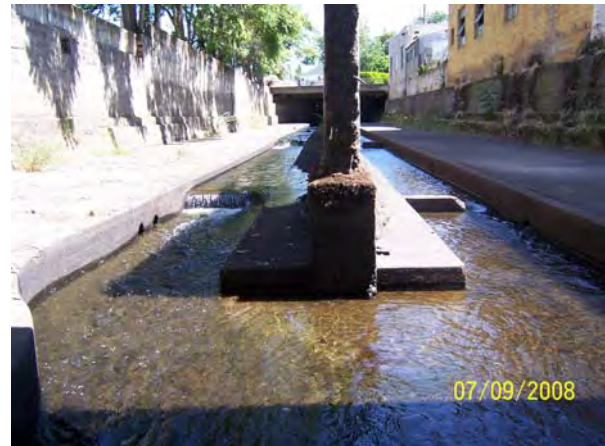
Photo 2.6 - Typical Reach Type 7 Split Flume with Center Wall. Flow is 6 cfs. View Upstream.
