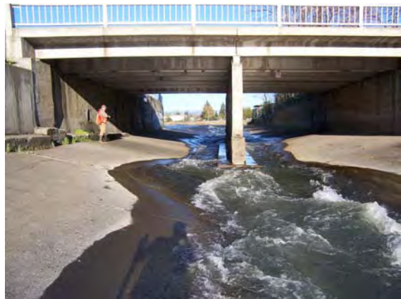
Photo 2.4 - Reach Type 4 Split Flume (Bridge Pier) at 180 cfs. View Upstream.
