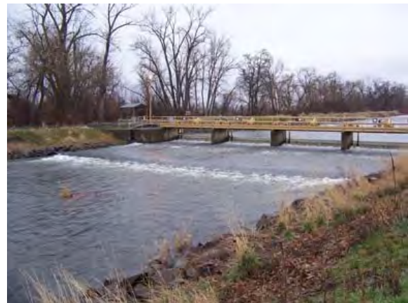
Photo 2.11 - Reach Type 12 Division Dam. Flow is 150 cfs. View Upstream.
