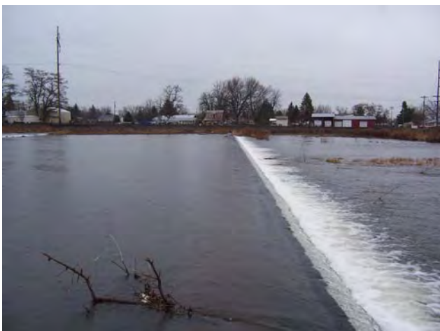
Photo 2.1 – A 200 foot long Reach Type 1 Sill at 208 cfs.
