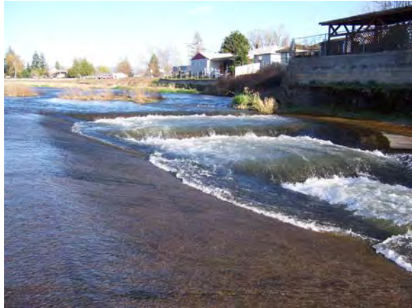
Photo 2.9 - Reach Type 11 Transition Fishway. Flow is 150 cfs. View Upstream.
