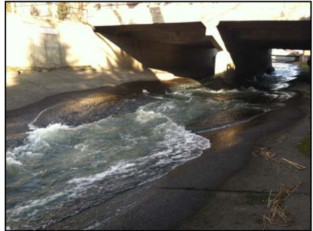
Figure 10 – View Upstream N. 5 th Ave Bridge.
