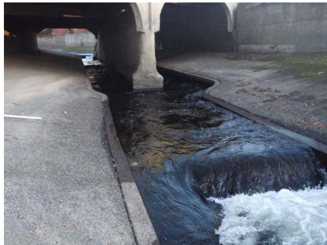
Figure 6 – View Upstream of the N. 6 th Ave Bridge Pier at 25 cfs.
