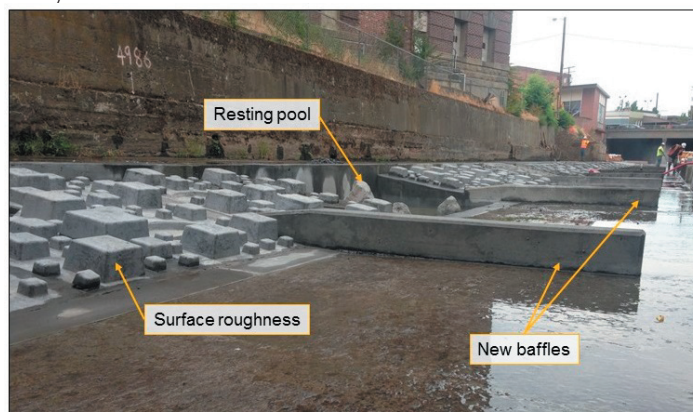
The proposed conditions for the Mill Creek channel. Roughness provides slower water favorable for adult passage. The new baffles improve juvenile passage during summer low flow.
