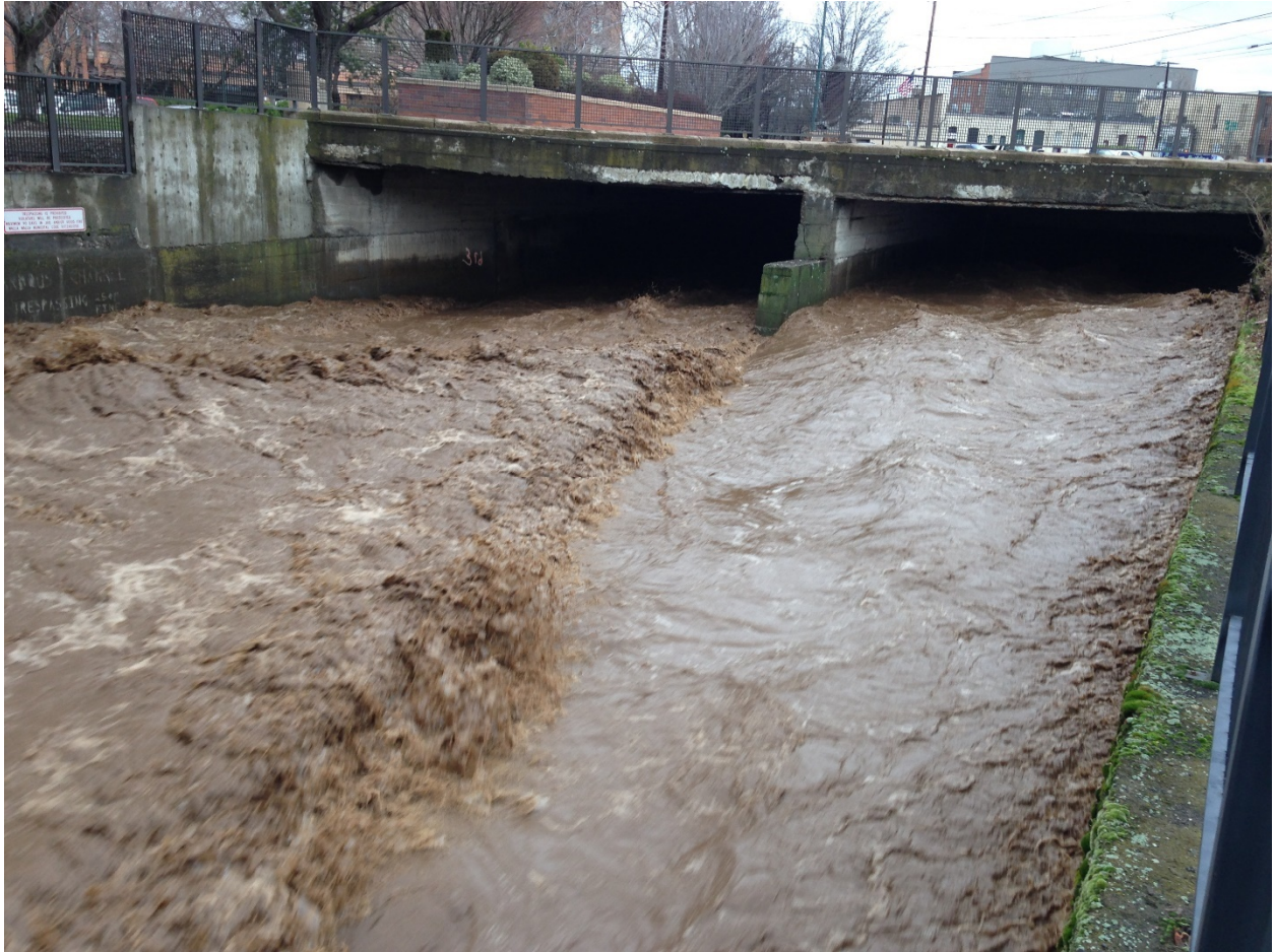
Figure 7 February 7, 2020 flooding looking up stream at the 3 rd Avenue Bridge and the underground. Flow is approximately 4000 cfs.
