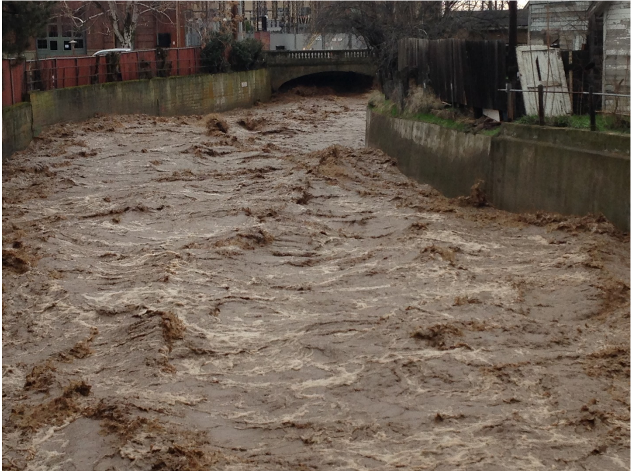
Figure 10 6th Avenue Bridge looking downstream from the 5th Avenue Bridge toward the start of the project.
