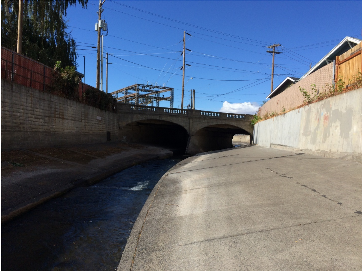
Figure 6 6th Avenue Bridge looking Downstream
