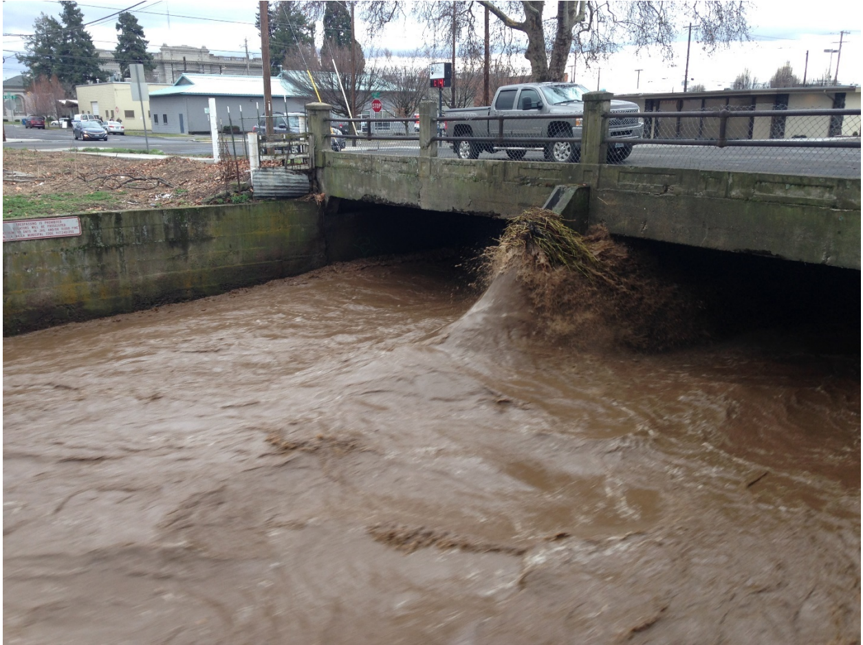
Figure 9 5th Avenue Bridge during 4000 cfs flows.
