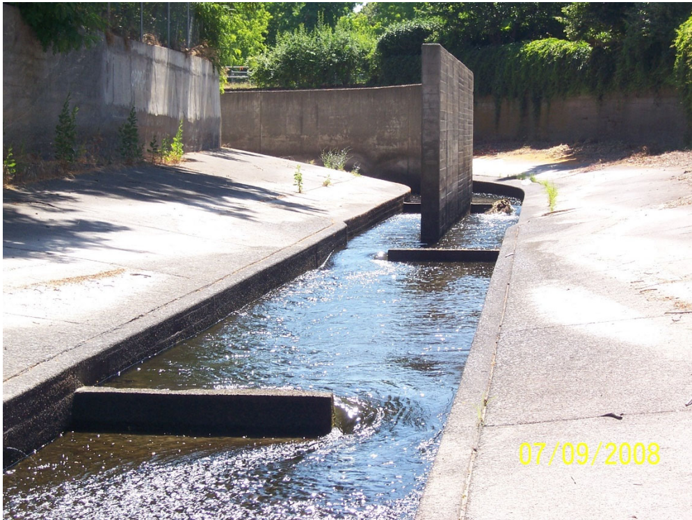
Photo 5 – View downstream of Reach Type 7 with sloping overbanks showing upstream end of wall and debris line. The foot bridge in the background is Marcus Street.
