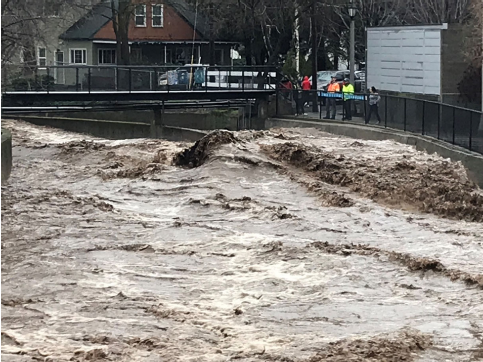
Photo 6 – 3500 cfs View of center wall with Marcus Street Footbridge in background.
