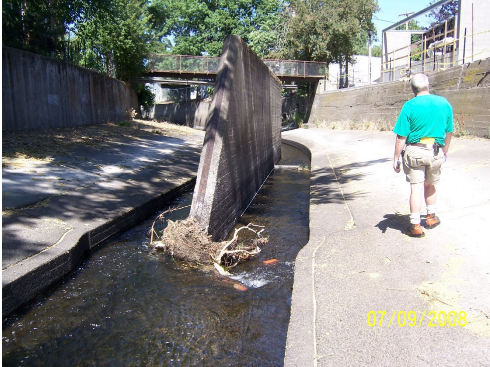
Photo 5 – View downstream of Reach Type 7 with sloping overbanks showing upstream end of wall and debris line. The foot bridge in the background is Marcus Street.
