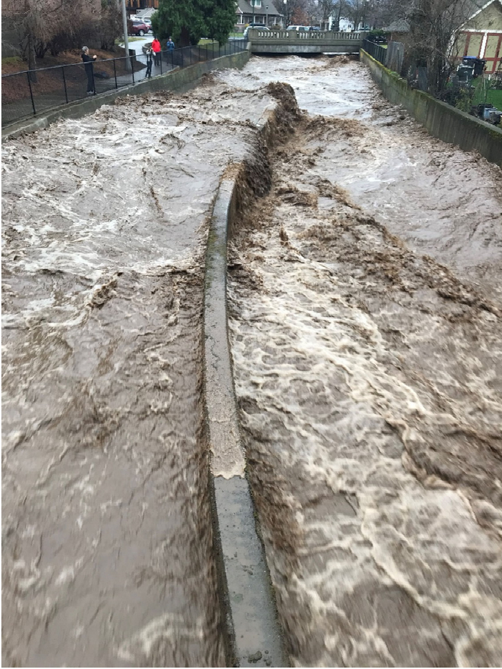
Photo 7 – 3500 cfs flow view upstream towards Park Street.
