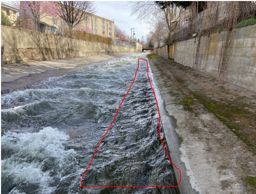
Photo 10 – View upstream showing roughness panel boundary layer. The velocity varies \pm 0.3 fps parallel to the flow due to the standing waves which form every 15 to 20 feet from the baffles across the channel.
