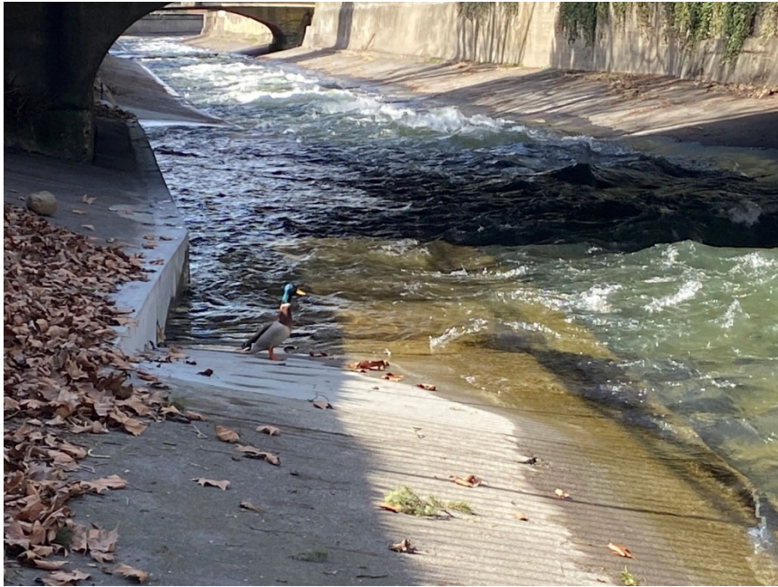
Photo 9 – View downstream of the Merriam Bridge. Unlike the typical Reach Type 3 Channel the left overbank (truck path) is submerged and carries a lot of water which reduces the effectiveness of the boundary layer. On average the velocities in the roughness panel are 0.5 fps higher than sections with no overflow.
